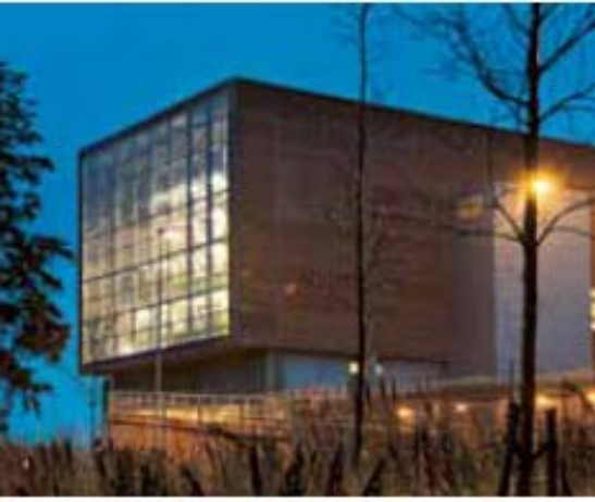
Unit 5 of the heating plant in Uppsala
