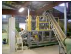
Nanshin Biomass Coop's pellet manufacturing plant
